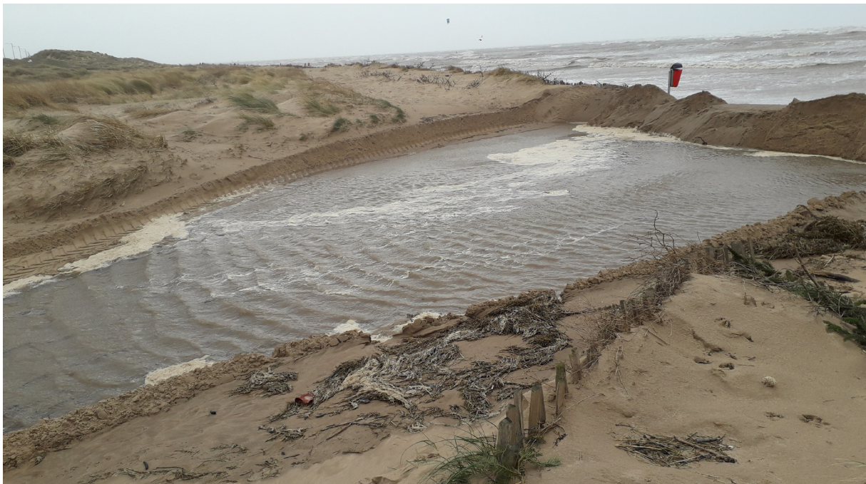
Storm Ciara and Storm Dennis Dunes Damage Feb 2020 - High Tide at NBCP Entrance
