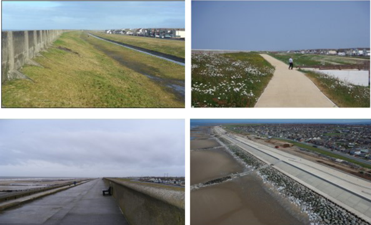
Figure 13: Rossall Coastal Defences Before & After
